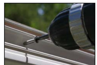
Fasten screen base (Stagger fasteners along left and right edges)
